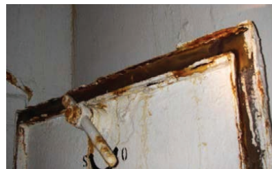
Corroded packing
