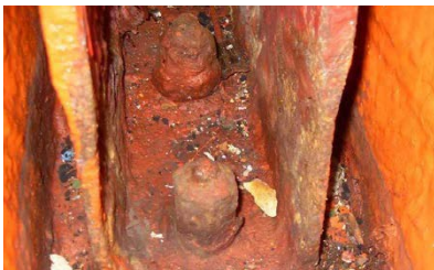
Wasted support bracket
